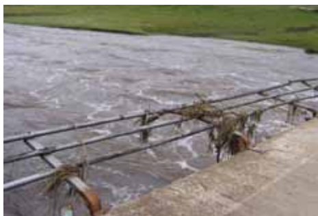
The power of water flattened these railings on MT01. Photo: Colin Williams.
